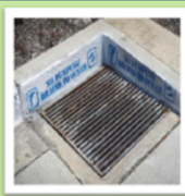
Storm drain inlet on private property
