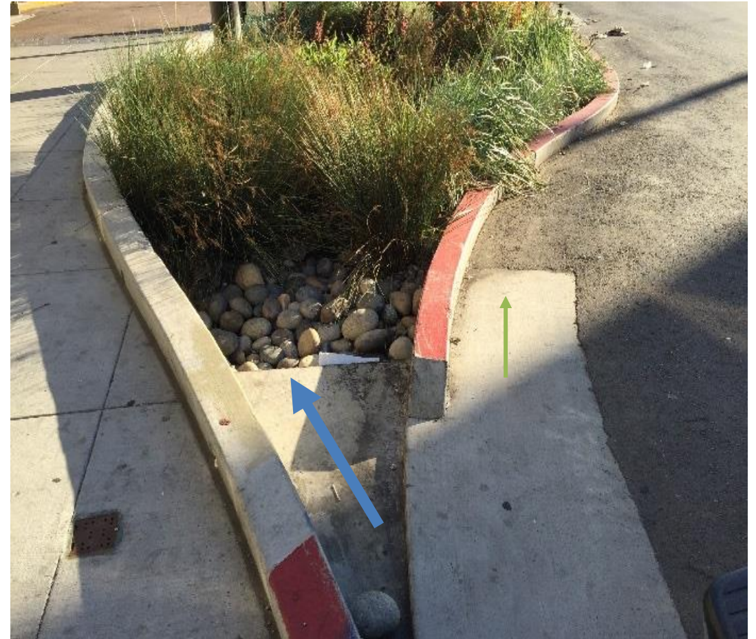
In-line design with Splash Apron and Cobbles
