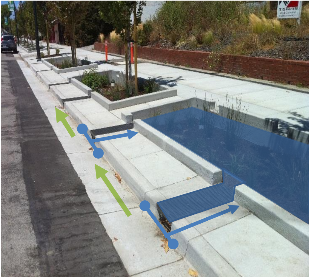
Off-line design with trench drains & wood mulch
