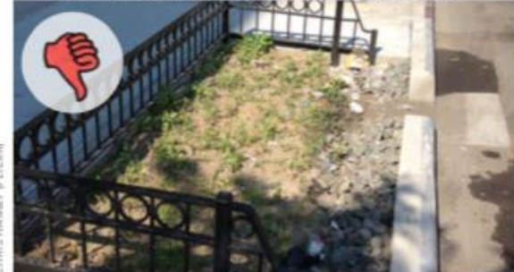
Poor, Overhaul Maintenance Routine
