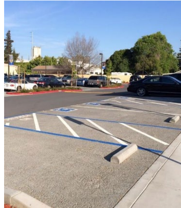
Pervious Concrete Parking Stalls (San Jose, CA)
