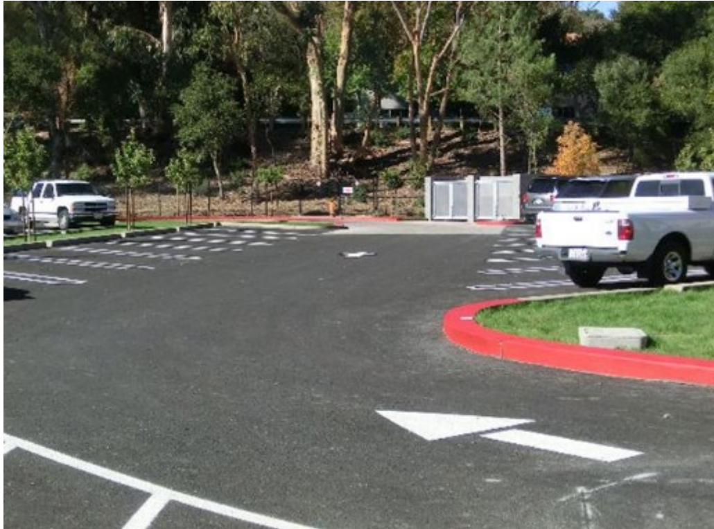
Pervious Asphalt Parking Lot (Los Gatos, CA)
