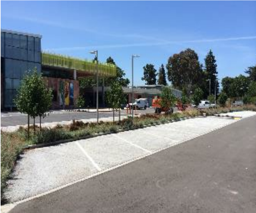
Tree Well Filter
