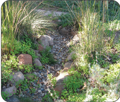
Dry creek infiltrates and conveys runoff.
