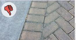
*Condition:* Excessive build-up of sediment inhibits infiltration between pervious paver joints.
