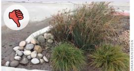
*Condition:* Sediment build up is severe enough to impede flow and inhibit landscape infiltration.
