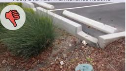
Condition: Little or no provisions for erosion control at curb cut entries.
