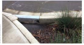
*Condition:* Sediment build up is occurring but not yet impacting the flow of water entering the landscape.
