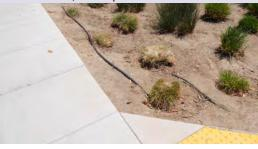
Condition: Irrigation lines/valves are exposed and prone to damage and/or vandalism.
