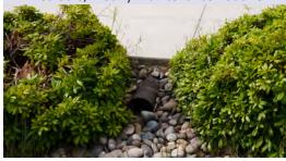
Condition: Curb cuts have some erosion control measures, but are still prone to erosion.
