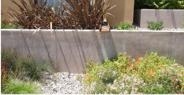
A roof downspout uses a metal channel to direct roof stormwater into a planter area. It is critical that the planter maintains a rock mulch or concrete splash pad to dissipate the vertical energy of water spilling into the landscape area.
