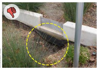
A Without a hard splash pad, the soil downstream of this weir is experiencing significant erosion.
