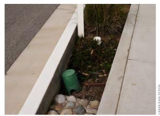
A green street with exposed drip irrigation lines and valve box is very susceptible to breakage.
