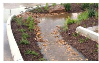
▲ Smaller rock at the flow line of a vegetated swale reduces to potential of erosion.
