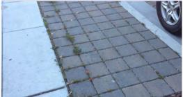
*Condition:* Some pervious paving joints are beginning to fill with sediment and debris slowing infiltration.
