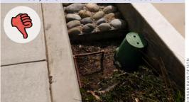
Condition: Irrigation system components are damaged/compromised due to exposure and damage.
