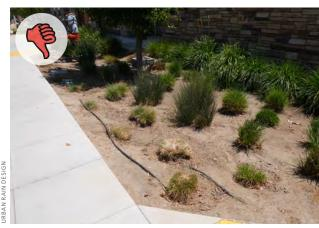
▲ A rain garden without regular mulch replacement results in plant desiccation and exposed drip irrigation lines.
