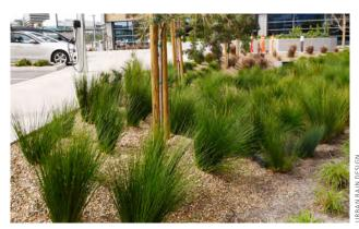
▲ Pea gravel mulch used on both the side slopes and wetted area of a vegetated swale prevents erosion.
