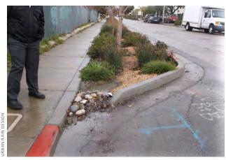
A River rock used to minimize erosion inhibits flow and creates sediment accumulation that is difficult to remove.
