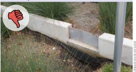
*Condition:* No splash pad is present causing severe erosion at water flow point.
