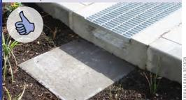
Condition: Splash pad at water flow point is adequately controlling erosion.
