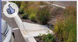
Condition: Curb cuts are properly graded and armored for erosion control.
