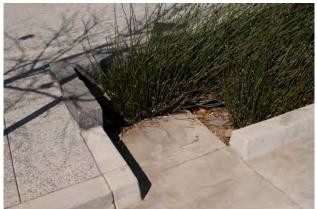
This stormwater planter features a concrete sediment forebay that can be cleaned easily using a flat-bed shovel.
