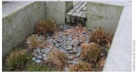
Condition: Water flow point only uses piled rock as a splash point. Some signs of erosion/rock movement.
