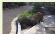
▲ This stormwater curb extension has a concrete forebay that captures sediment that is removed regularly.
