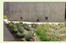
▲ This rain garden at the UC Davis campus captures roof runoff and features drought-tolerant plantings.
