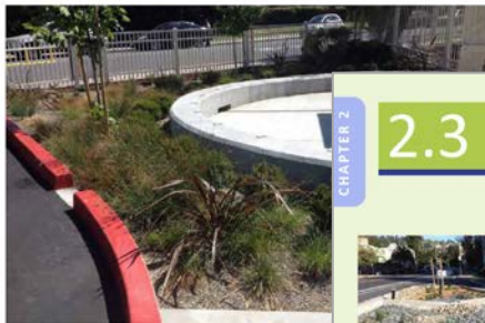
▲ A rain garden capturing surface and roof runoff at Laurel Elementary in San Mateo County.
