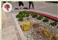
▲ Commonly, this stormwater curb extension inlet rim is fixed at the chain grade of rock mulch leaving little opportunity for water retention.
