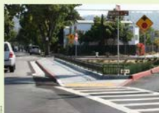
▲ An offset and angled intersection was retrofitted to include an extensive rain garden. Storm drain pipes from two streets runoff into the rain garden, which set the design of the rain garden.
