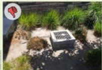
▲ The storm inlet rim is fixed at a height of over 8 inches. If this rain garden does not infiltrate or a manhole cover is installed, it could cause the effects of too much prolonged standing water.
