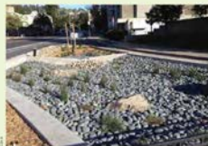
▲ Check dam slows runoff in sloped street canyons. This rain garden is also used to separate vehicles and bicycle facilities.
