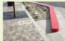
▲ While this is a good concrete pad, the elevation needs to be lowered at least 2 inches to allow for sediment capture.
