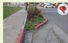
▲ This stormwater curb extension has no concrete forebay. Sediment build-up and blocks runoff from entering.
