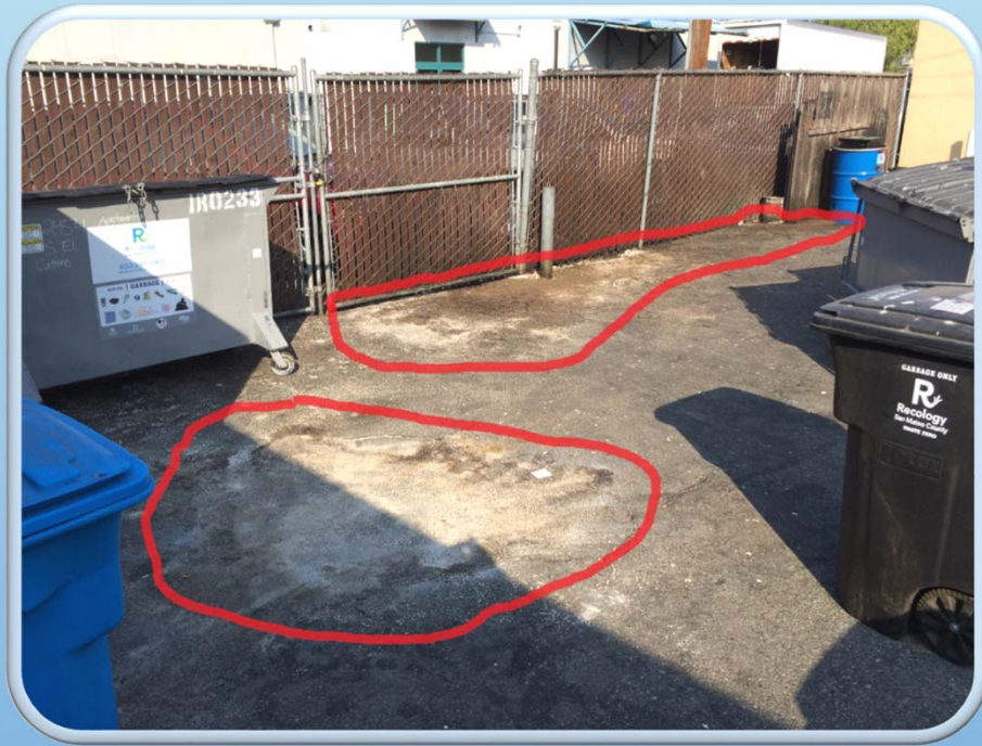
Areas of asphalt affected by oil saturation
