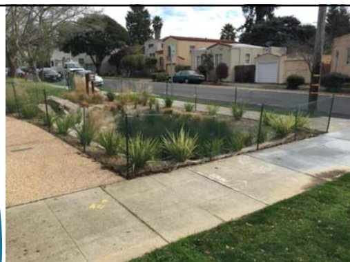
After: re-graded area with new rain garden treating street run-off
