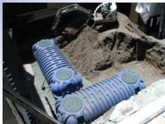
Cisterns installed underground
