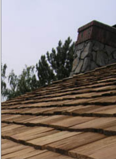
Wood shingle roof Courtesy of Gutter Glove
