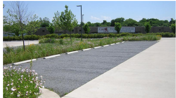
Figure 2-38: A plastic grid system filled with gravel provides the structural strength for a vehicle to slowly drive on.
