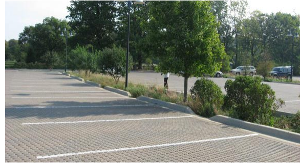
Figure 2-43: Pervious joint pavers within a parking lot application. Any overflow from the pervious pavers drains into a swale.
