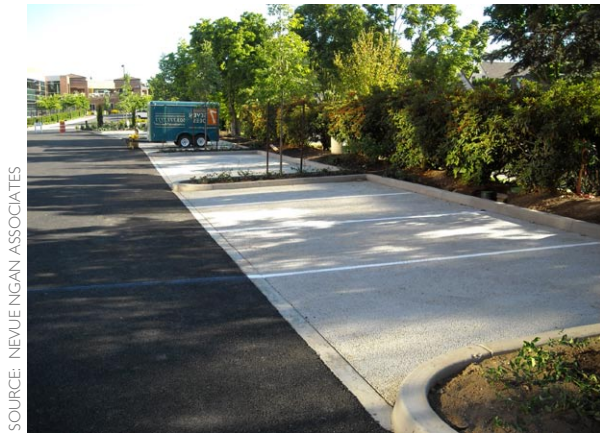
Figure 2-41: Pervious concrete allows for stormwater management and its light color helps reflect heat rather than absorb it.
