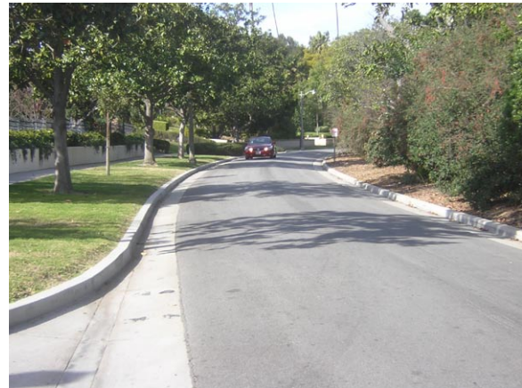
Figure 2-3: This narrow residential street maximizes the amount of landscape space and minimizes the amount of impervious area that generates stormwater runoff.
