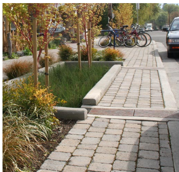
Figure I-24: This green street retrofit project in Portland, Oregon was built not out of a requirement, rather it was built simply because it could be done.
