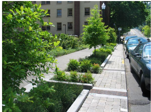
Figure 6-4: SW 12th Avenue Green Street in Portland, Oregon is another downtown green street project that was built inexpensively because it did not impact the existing piped infrastructure.
