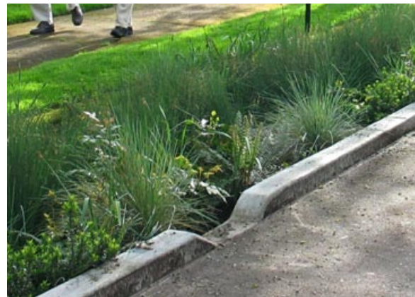
Figure 6-10: In contrast to the example above, a simple cost-effective curb cut allows water to move freely into a stormwater facility without detracting from the aesthetics of the project.
