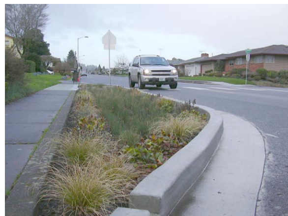
Figure 6-11: This mid-block stormwater curb extension project keeps the existing street curb in place and allows stormwater runoff to overflow back into the street without using any piped overflow structures. The combination of these strategies helped reduce construction costs.
