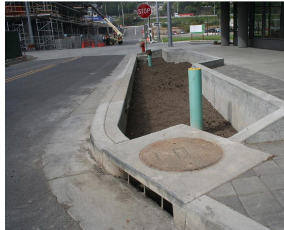
Figure 6-9: This high-cost, engineered green street example uses a lot of concrete infrastructure, as well as uses an inlet structure that makes stormwater appear to be a waste rather than a resource.
