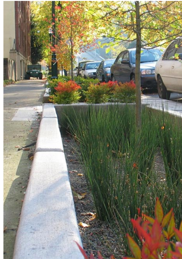
Figure 5-57: A 2 inch layer of pea gravel mulch is applied within a stormwater planter.
