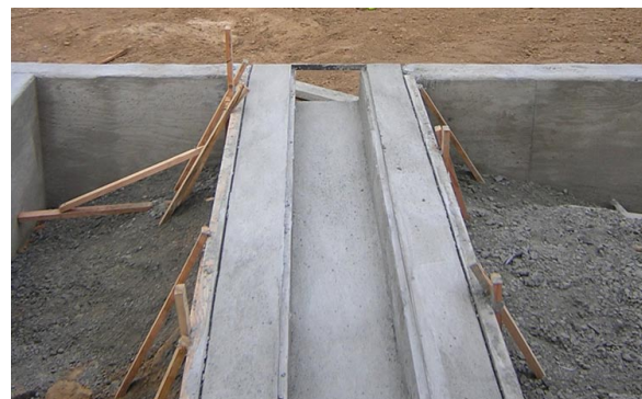
Figure 5-55: Hardscape elements, such as this trench drain channel, should be inspected to ensure positive drainage into the stormwater facility.
