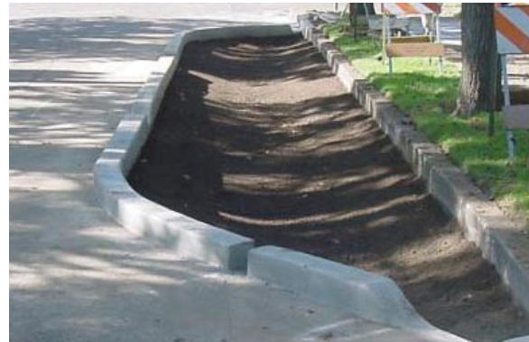
Figure 5-54: A shallow graded stormwater curb extension retains a maximum of 7 inches of water.
