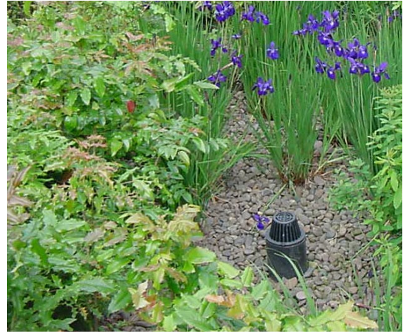
Figure 5-44: Overflow from this rain garden enters a 6 inch riser connected to the storm drain system.
