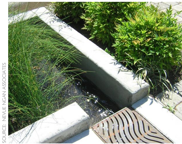
Figure 5-41: A small, 18 inch wide sediment forebay at the entry curb cut of a street stormwater planter.
