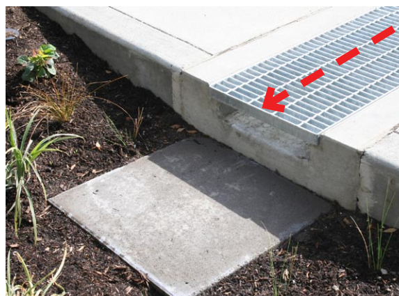
Figure 5-38: A concrete unit paver is placed at the exit point of this trench drain. The pad helps prevent erosion by dissipating water velocity as water drops from the trench drain to the finish grade of the stormwater facility.
