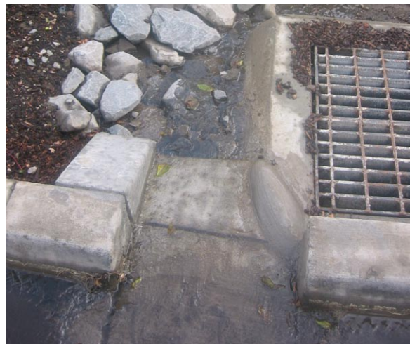
Figure 5-30: Bad example - a curb cut placed immediately adjacent to the overflow inlet.
