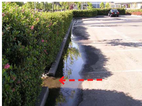
Figure 5-31: Bad example - a curb cut blocked by sediment prevents water flow into this stormwater facility. There is not enough grade change between the curb cut entry and the finish grade of landscaping.
