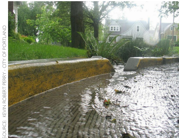
Figure 5-27: A typical curb cut used to allow water to enter a stormwater curb extension.
