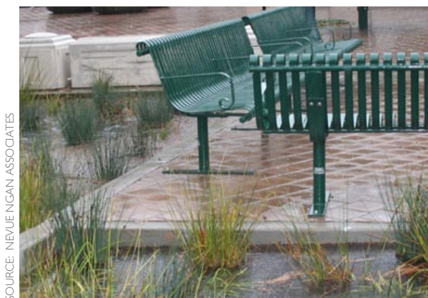
Figure 5-28: Sheet flow of stormwater runoff enters a vegetated swale from a public plaza space.
