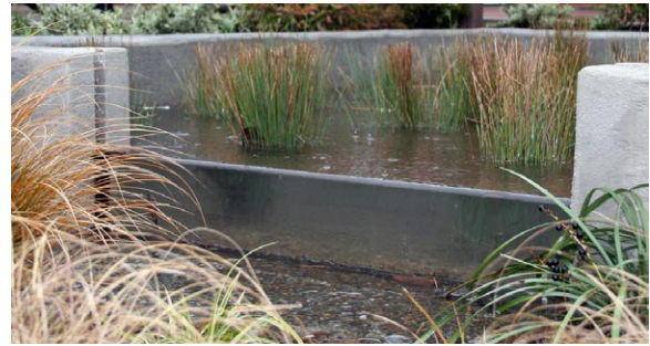
Figure 5-19: This adjustable weir can control how much water is to be retained within a rain garden.
