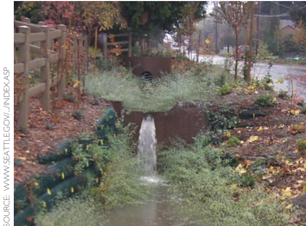
Figure 5-17: Terraced concrete weirs allow for a vegetated swale to be graded with a slope less severe than the adjacent street's grade.
