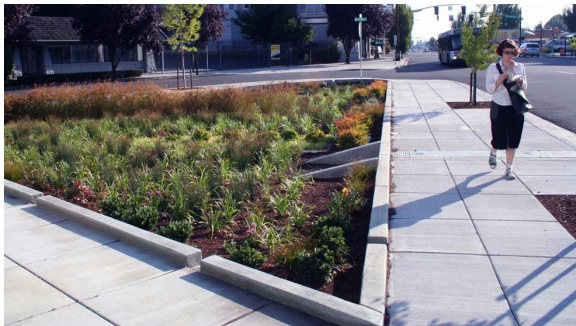
Figure 5-12: A perimeter concrete curb was installed around this urban rain garden to help protect both pedestrians and the stormwater facility.
