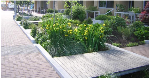
Figure 5-11: A series of “stormwater bridges” allows people to cross over a vegetated swale.
