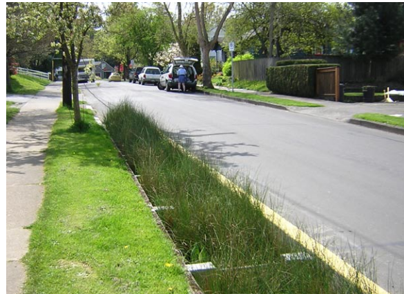
Figure 5-8: This green street retrofit is designed with a narrow curb extension that captures runoff from an existing crowned street.
