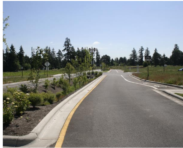
Figure 5-7: This newly constructed green street is designed as a reverse-crowned street, allowing runoff to flow into a center median vegetated swale. In the example above, stormwater runoff enters the swale through inlet pipes. A better design solution would be for the runoff to enter on the surface via curb cuts.
