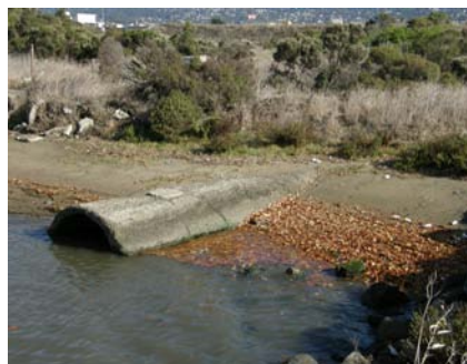
Like many of the creeks around the Bay, Schoolhouse Creek enters the Bay in a storm drain pipe. Photo by Lisa Owens Viani.
