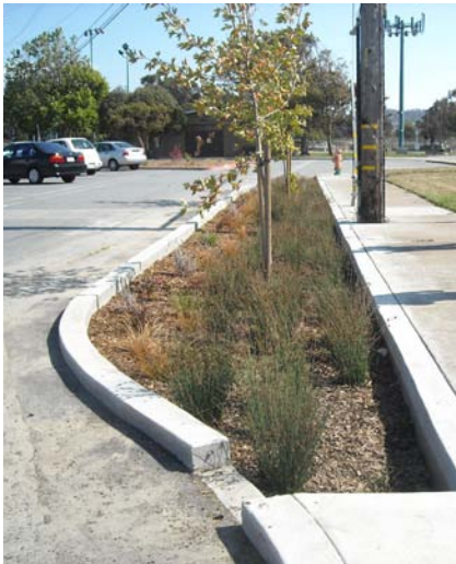
A curb extension in San Bruno (notice the cut in the curb). Photo courtesy San Mateo County.
