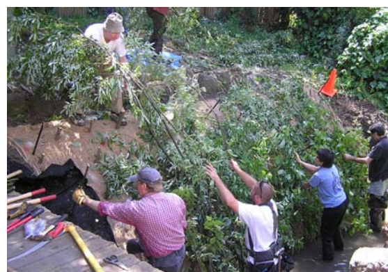
“Soil bioengineering” is a way to stabilize and green creek banks using plant material instead of riprap. It helps make our watersheds more resilient. Photo courtesy of Urban Creeks Council.
