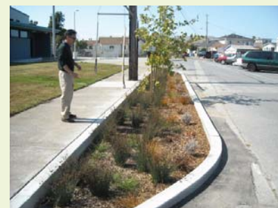
The design for the Belle Air/Third Avenue "street creek" project was featured as an example project in the San Mateo County Sustainable Green Streets and Parking Lots Design Guidebook.
