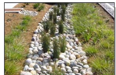
Bioretention system in Burlingame
