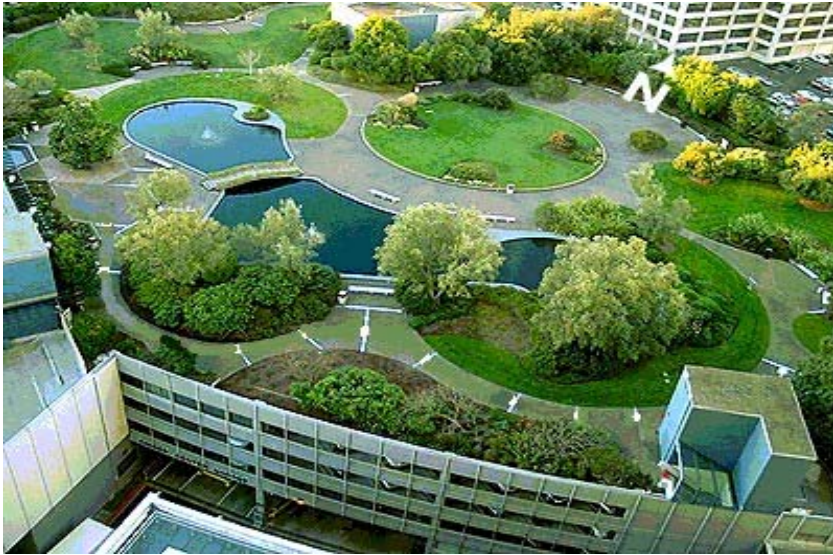
Figure4-9: Intensive Green Roof at Kaiser Center Parking Garage, Oakland.
